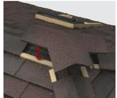
Fix rafter cap and ridge
